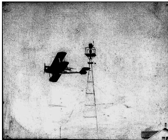
Figure 4. Wann, Nebraska (Dewell photo)—mail plane in flight. (Note object above lamp housing is a red light indicating no landing strip or conditions not adequate for landing.)
