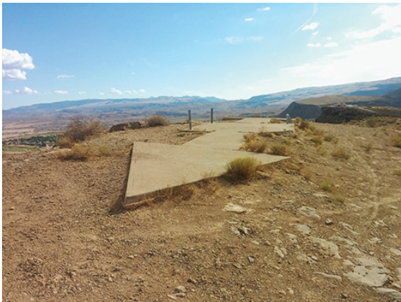
From Wikipedia, the remnants of Transcontinental Air Mail Route Beacon 37A, which was located atop a bluff in St. George, Utah. With concrete arrows indicating the direction to the next beacon, a rotating light tower, and a shed that usually held a generator and fuel tanks, these beacons were once situated every 10 miles on air routes across the United States beginning around 1923.
